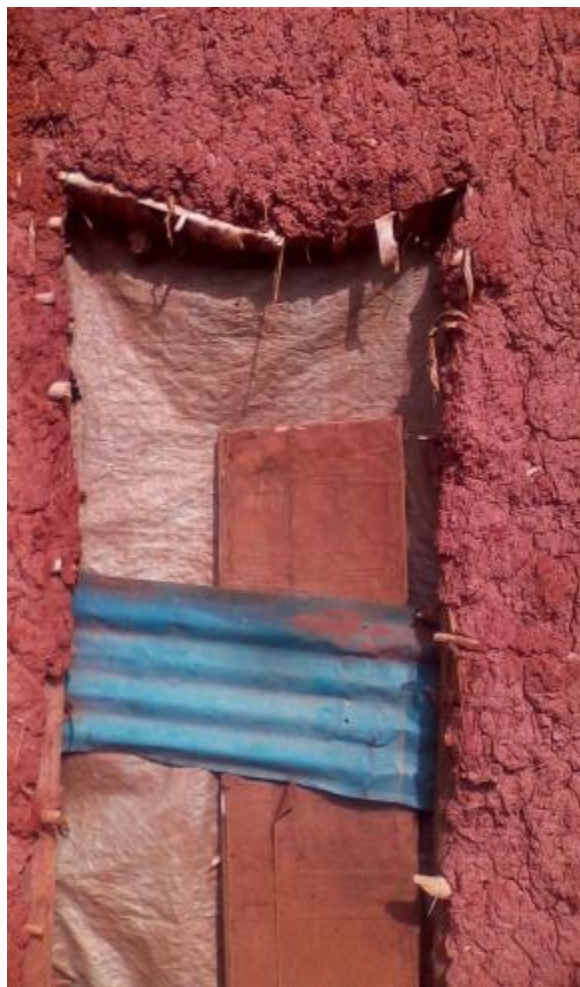
Picture 9: Door made of iron sheeting
